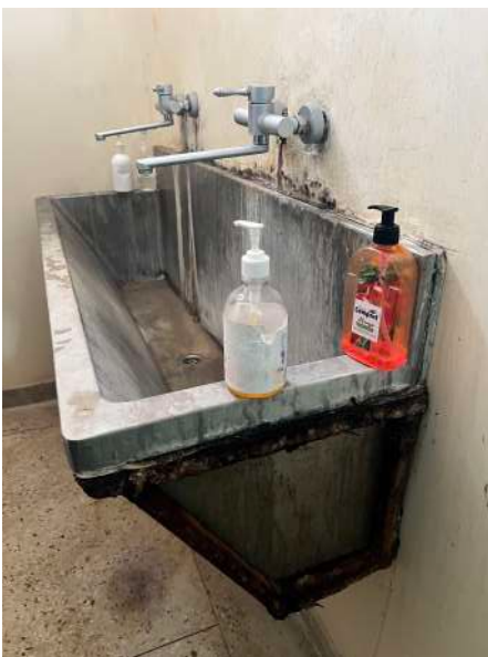
Scrub facilities in the theatre complex, with intermittent water supply
